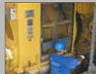
AME disassembled, cleaned, repaired and reassembled the unit in their shop. It was then shipped back to the Turks and Caicos, where an AME Service Engineer supervised the install, did a laser alignment, and a Windrock Survey of the engine.
